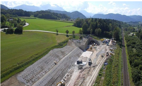
Tunnel Stein Ostportal
