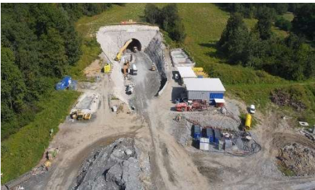
Tunnel Lind Westportal
