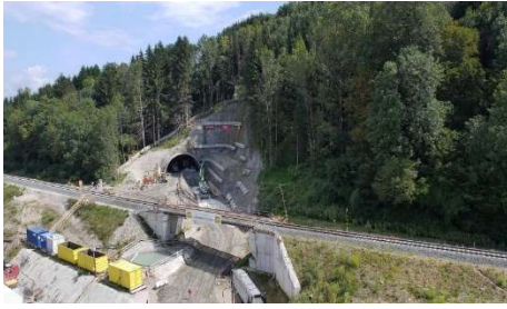
Tunnel Stein Westportal
