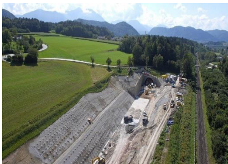
Ostportal Tunnel Stein
