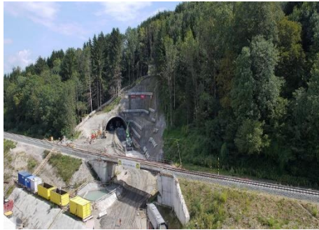
Westportal Tunnel Stein
