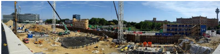
Monitoring HBF Wien Baustelle Parkhotel am Belvedere
